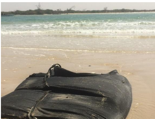
Photo 6: Seawall protection with sandbags, destroyed after a surge. Sambou D. 01/2019
